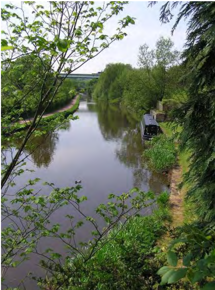
Photo. 39 Leeds and Liverpool Canal towards Gathurst Bridge and M6 Viaduct.
