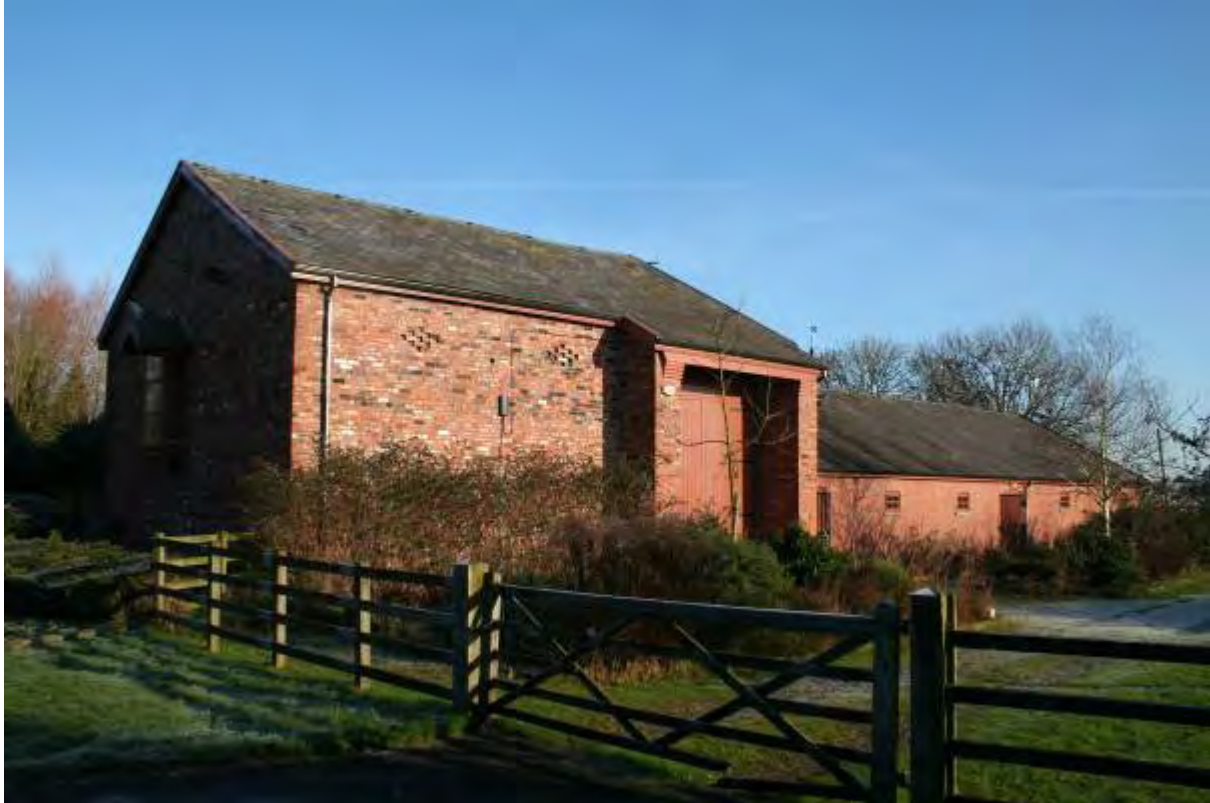
Photo 175 Hope Carr threshing barn / Interpretative centre.
