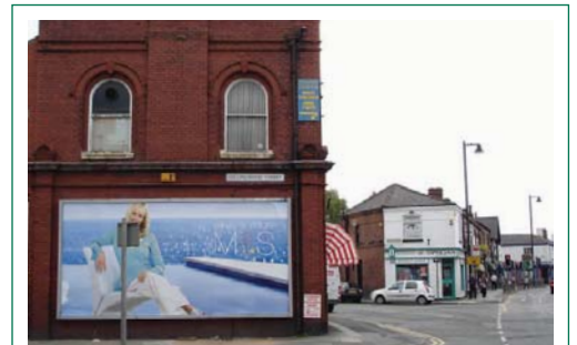
This large poster may be authorised but its scale is excessive in relation to its host building.
