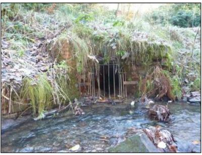
The entrance consists of two brick pillars supporting a large concrete slab over the brick archway of the drain itself. An iron grille has also been fitted across the opening. The entrance is in reasonable condition; some of the bricks on the right-hand side of the arch have slightly deteriorated but are stable. Vegetation has grown over the brick pillars and concrete slab.
