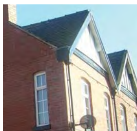
mortar verge detail
