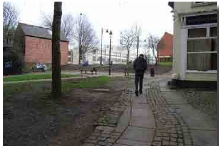
Old setts and flags will be retained and maintained as they contribute to the historic character of a street
