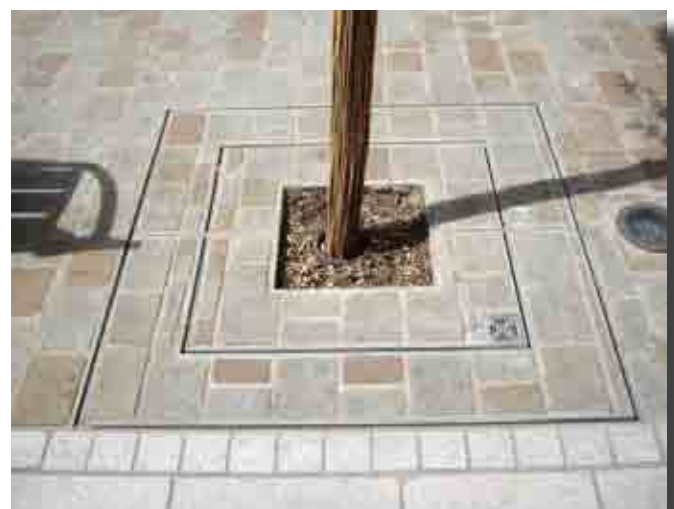
For ease of maintenance tree grilles should be either permeable resin bound tree pit mix or yorkstone
