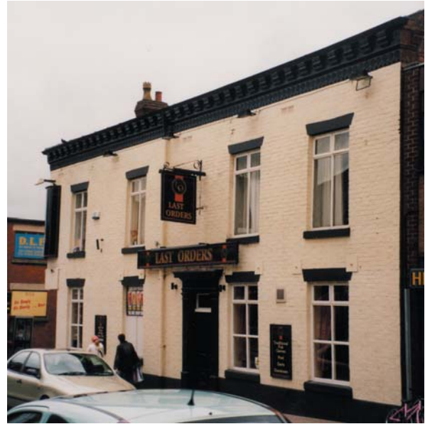
The Last Orders public house retains Doric doorcases and a heavily moulded brick eaves cornice.
