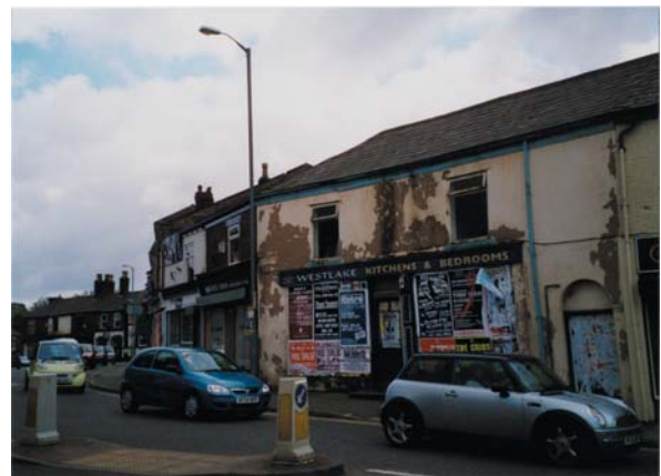
No.21 Market Street ‘AT RISK’.
