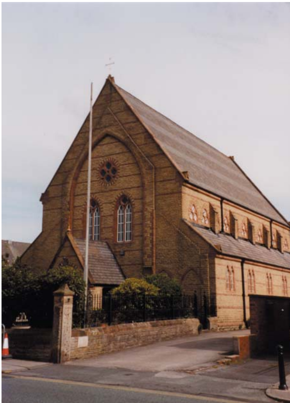
The Church of St Benedict has distinctive elevations of buff gritstone bonded by red sandstone designed by Joseph Hansom (1869).
