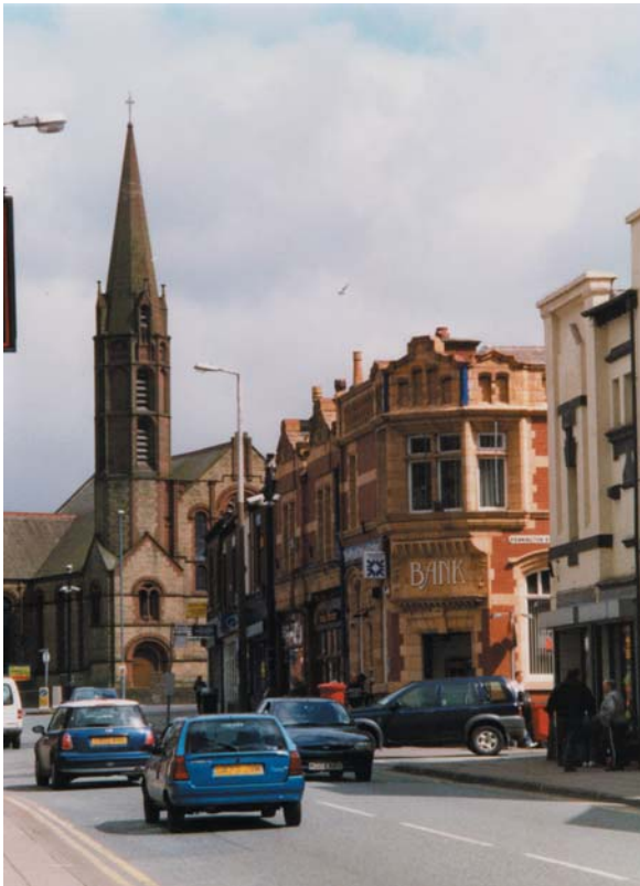
The elegant spire of St. John's Methodist Church provides an important focal point at the northern end of Market Street.
