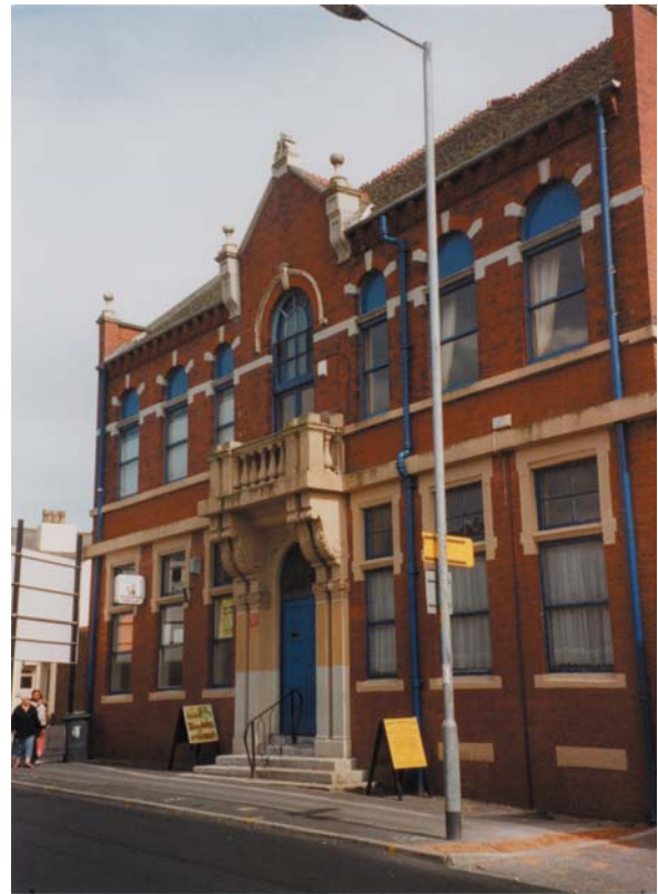
The Conservative Club, No.135 Market Street has a grandiose doorcase and imposing scale.
