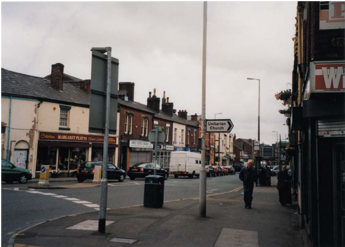
The public realm at the northern end of Market Street is cluttered and unco-ordinated with low quality surface finishes.
