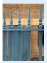
This is a simple fence constructed from galvanised tubular steel which is welded to both the upper and lower horizontal bars. The fence can be customised and made more ornate by the addition of a wide selection of finials. It is attractive and inexpensive and offers a good level of visibility.
