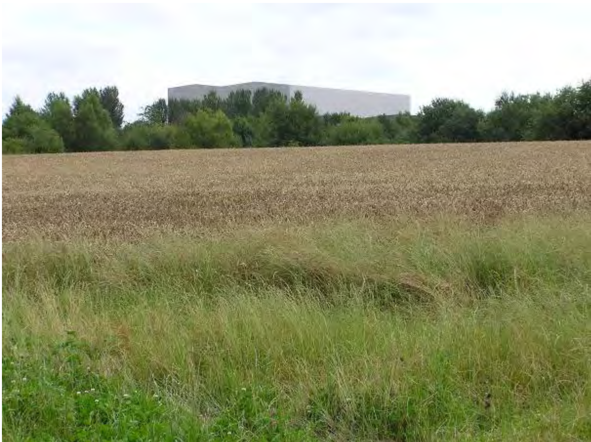
Photo. 121 A view of part of the Heinz Factory from fields just north of Crooke.
