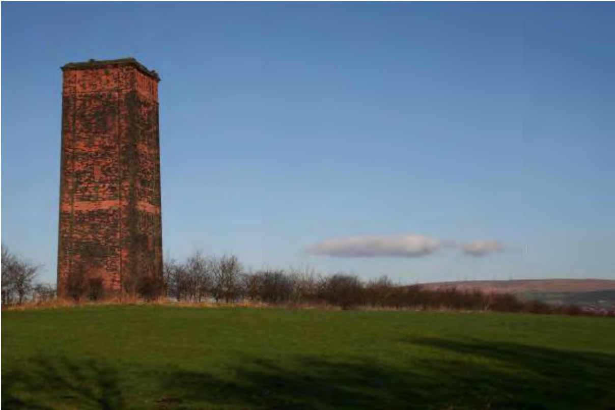
Photo 143 Wall Hey Pit Ventilation Shaft, Haigh Road, Aspull.
