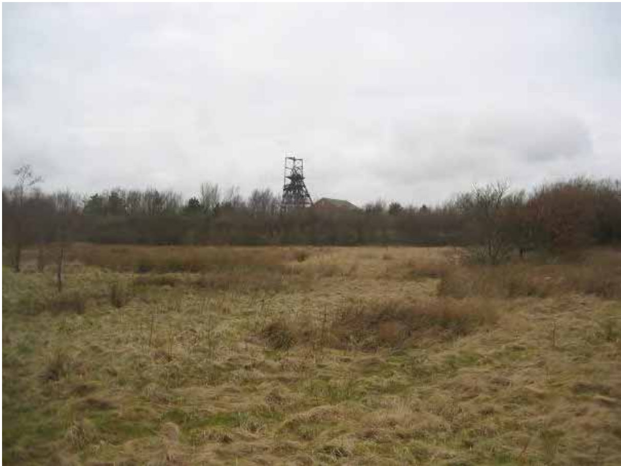
Photo. 1 Astley Green Pit winding gear.
