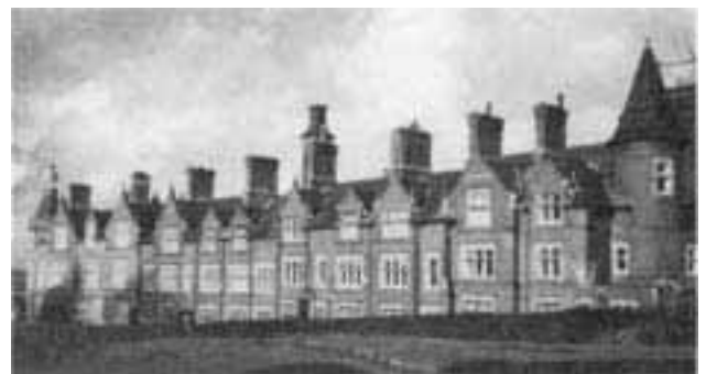
Gerrard Winstanley House and County Courts
