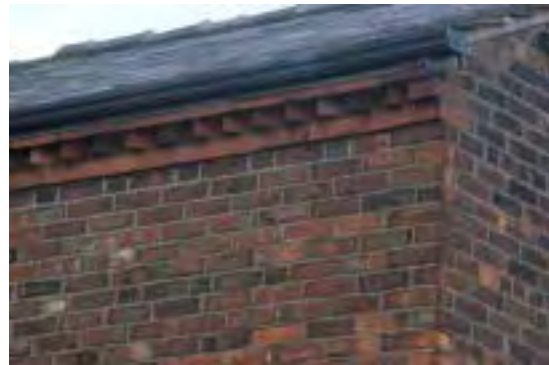
In many cases the differing eaves detailing could have been the individual builders mark and provide a simple variation and individuality.
