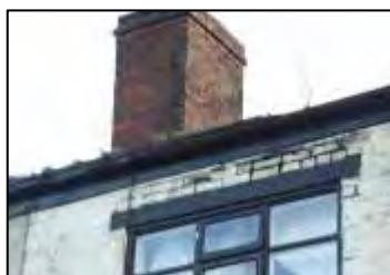
Photograph 38: Faulty guttering
