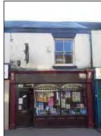
Photograph 20: Historic shop front at 14 Market Street
