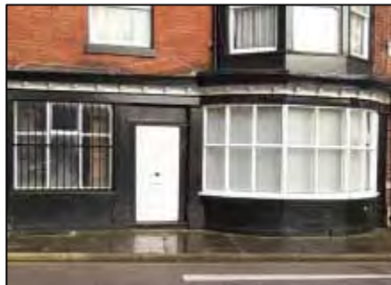
Photograph 18 (below): Historic shop front at 5 Market Place
