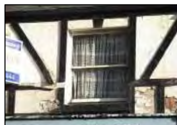
Photograph 40: Rotting wood
