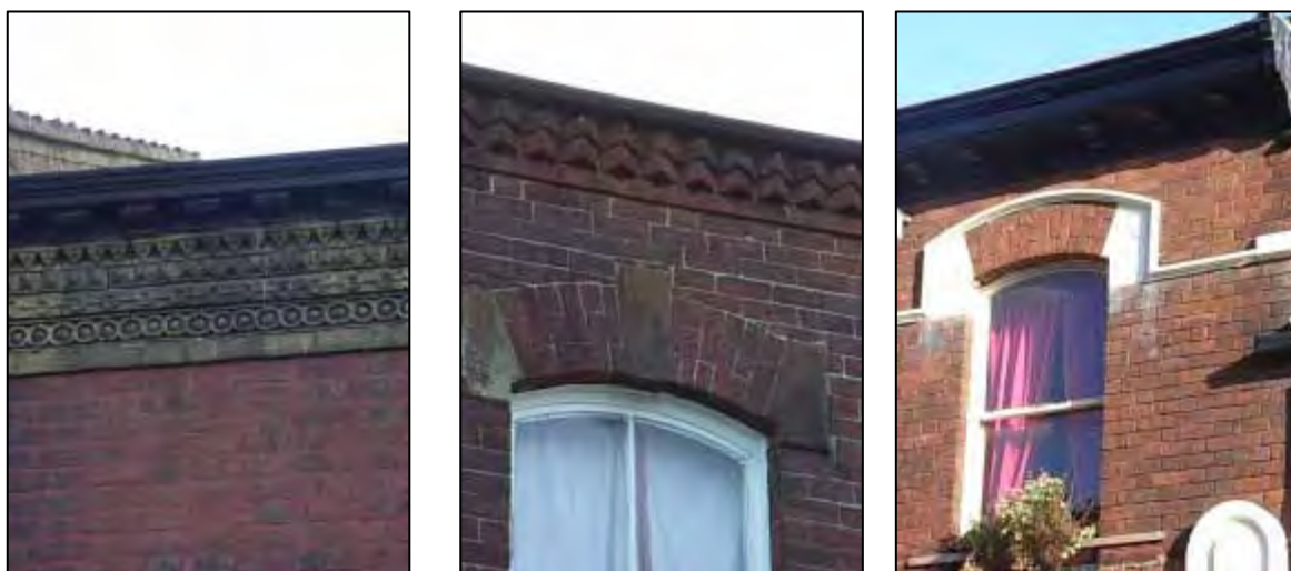
Photograph 8, 9 &10: Examples of Corbelling and window detailing
