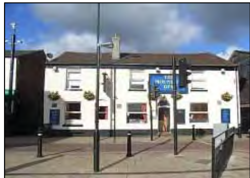
Photograph 30: Showing the detrimental effect overuse can cause to architecture.
