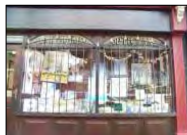
Photograph 47 (right): Decorative grilles on 14 Market Street
