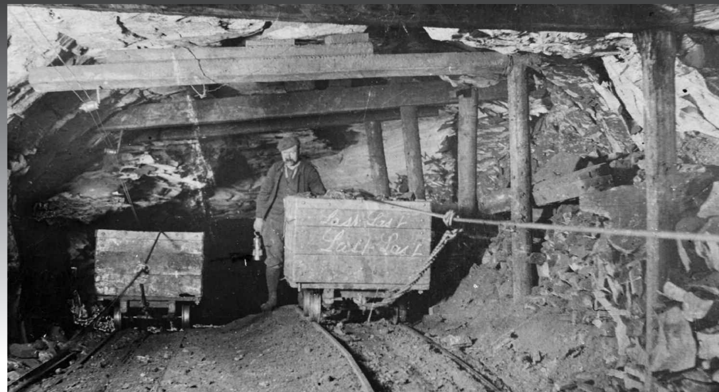
Coal haulage in tubs linked to a rope haulage system, Bamfurlong Colliery, Ashton-in-Makerfield, c. 1920
