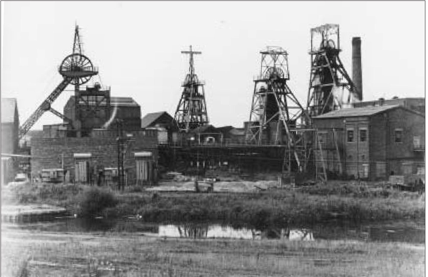
Cliff Reeves, of Parish Video, has sent in this splendid photograph of Bickershaw Colliery in the 1970's. The colliery opened 125 years ago, and closed 10 years ago.
