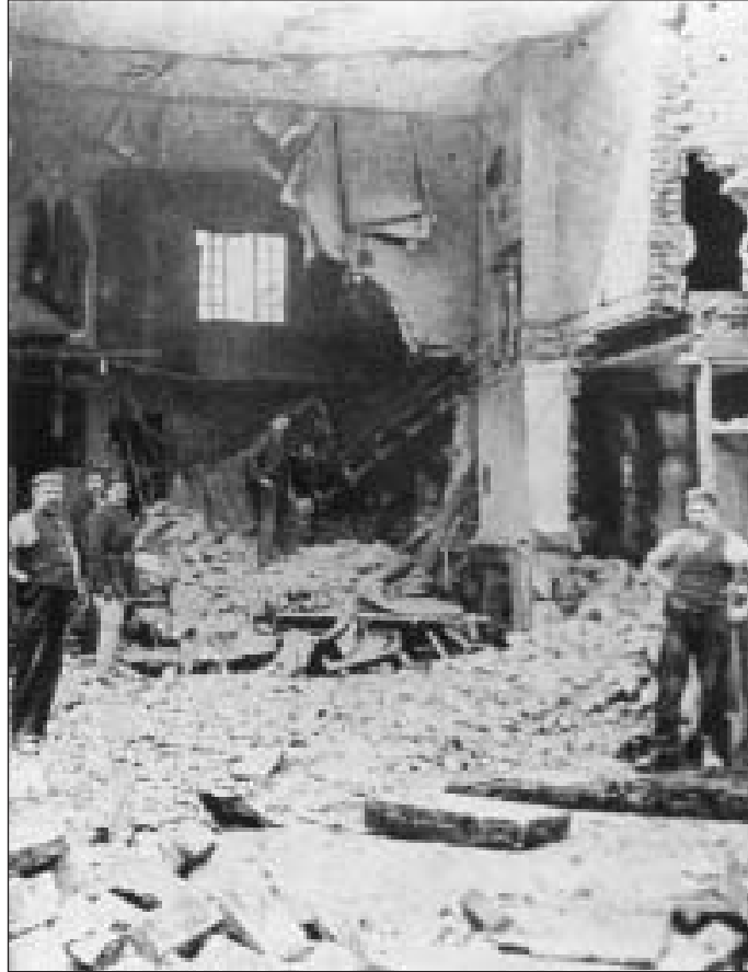
Gas Explosion at Leigh, 23 May 1905.
