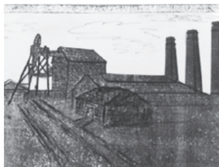
Button Pit, each of the three furnaces had a separate squat chimney; it was said that this construction was adopted so that it would not spoil the view from Haigh Hall
