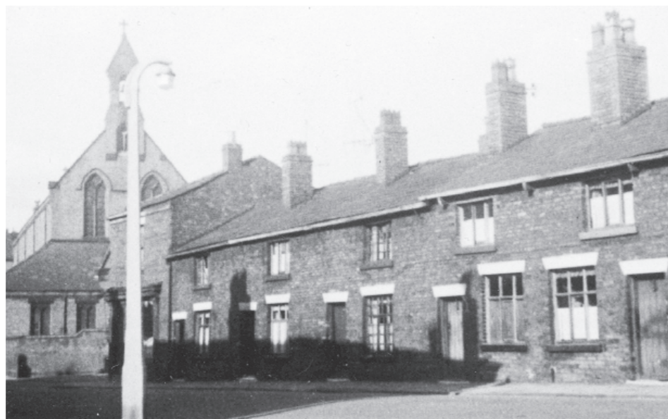
St Patrick's Church, visible behind cottages in Hardybutts
