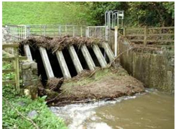
These screens themselves are often prone to blockage and require frequent clearance and robust emergency procedures in place to ensure that they do not in themselves cause, flooding.
