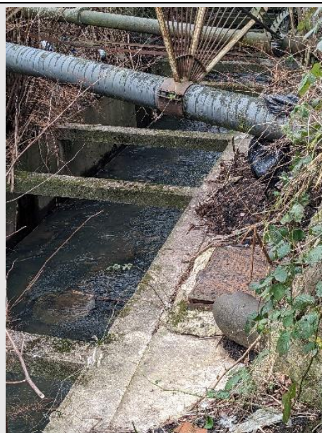
Photo 2: Highway drain outfall into Hey Brook (Source: JBA Consulting).
