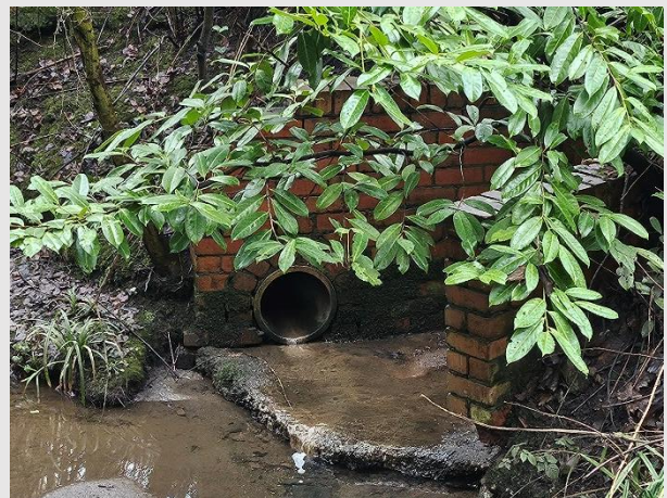
Photo 5: United Utilities surface water sewer which outfalls into Brookside Brook Drain. The Highway drain outfall is situated to the right (Source: JBA Consulting).
