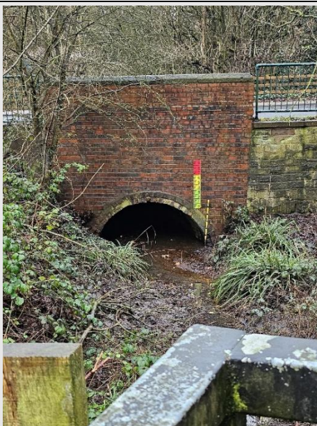
Photo 4: Culvert where Brookside Brook drain passes beneath Bickershaw Lane (Source: JBA Consulting).
