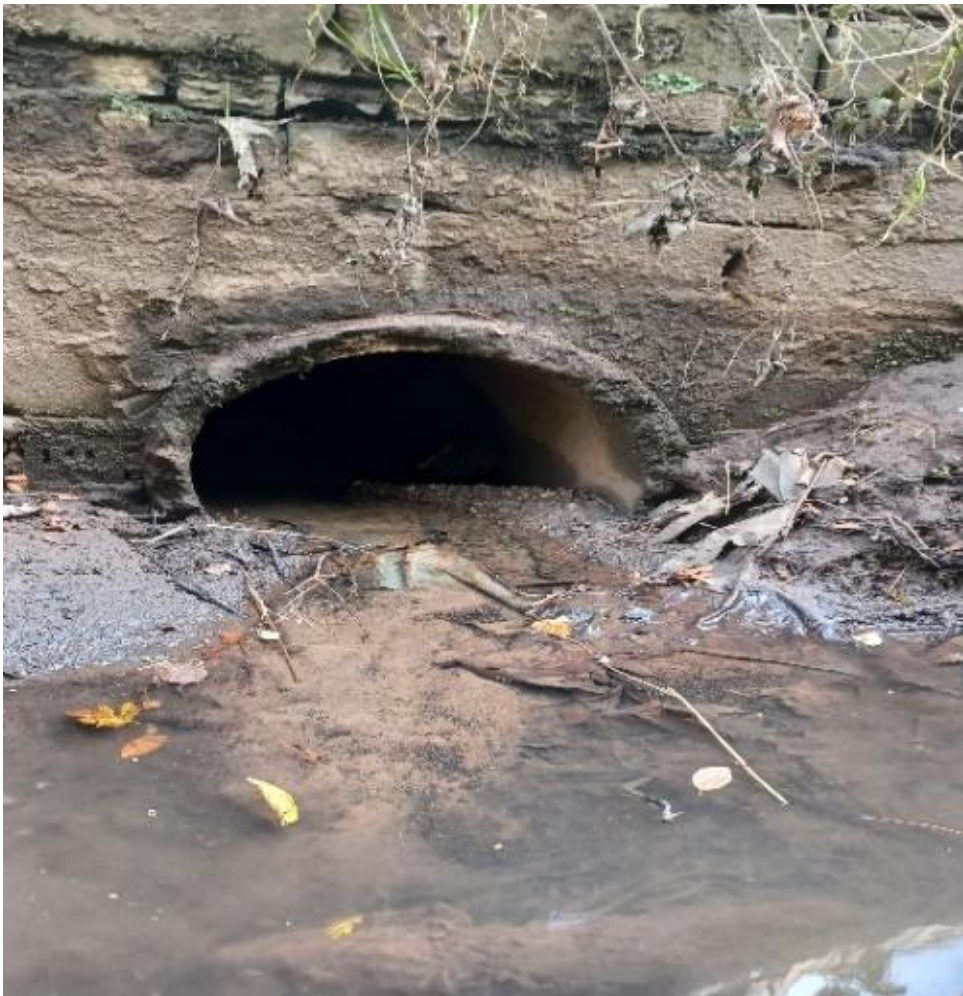
Figure 3-4: Photograph of outfall of culverted watercourse.
