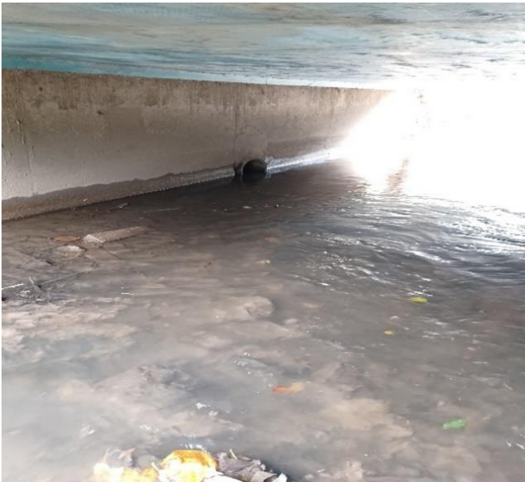
Figure 3-3: Photograph of outfall into the Millingford Brook from United Utilities' network.
