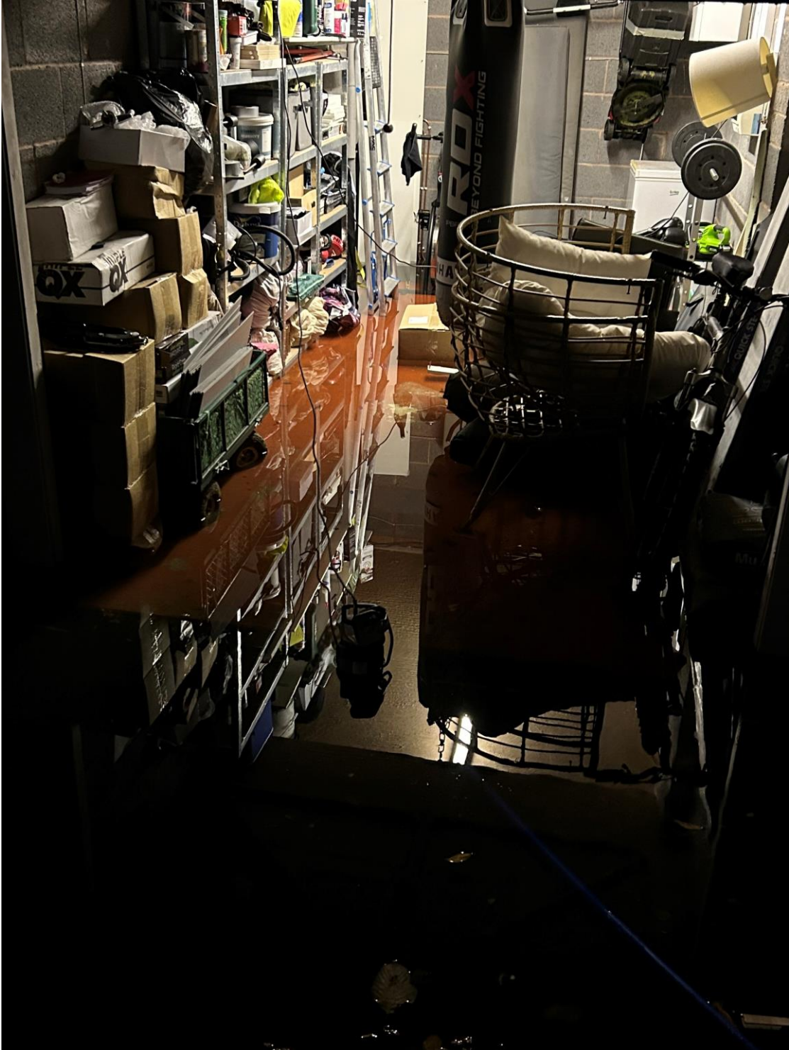
Figure 5 - Flooding to Property on May Tree Drive (Evening 06/11/2023)
