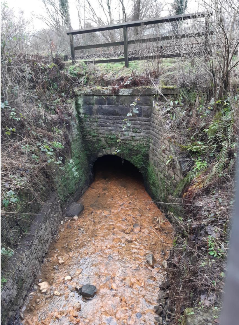
Figure 6 - Inlet to Network Rail Culvert Under Normal Conditions. Facing Downstream. Winter 2024.
