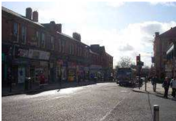
Photo 2.17a / b: Wallgate adjacent to Wallgate Railway station
