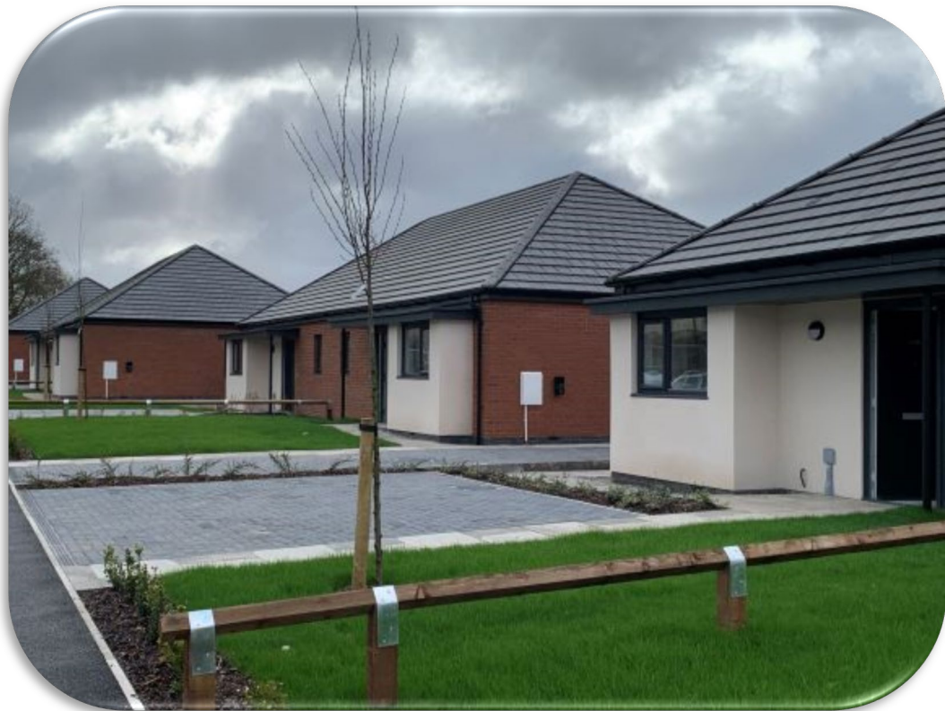
Picture: 8No. new build bungalows at York Street, as part of the Councils New Build Direct Delivery Scheme
