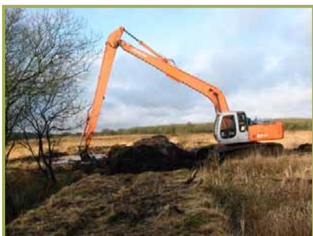
Bund heightening to isolate peat compartments
