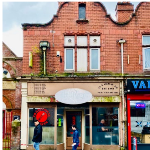
Poor condition and underinvestment in premises
