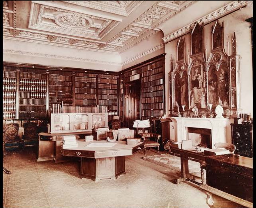
Haigh Hall, Library Ceiling Plaster
