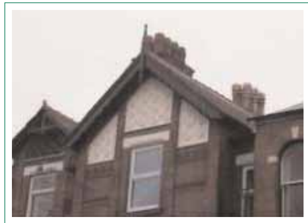
Detail of gable, No.16
