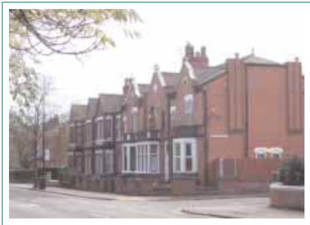
Nos 5-10 Park Road.
