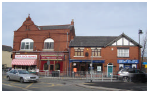
Figure STA.7: Pole Street
