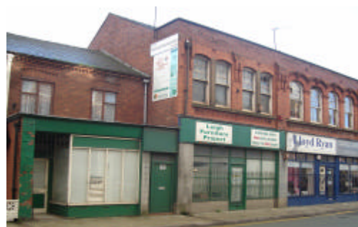
Figure TYL.9: Units on Elliott Street
