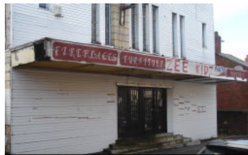
Figure TYL.4: Vacant Fireplace Warehouse
