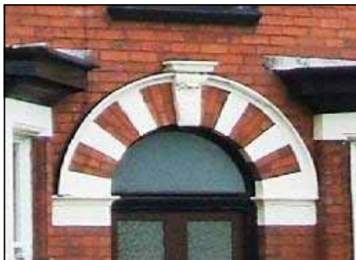
Photograph 10 (above): Detailed brick work
