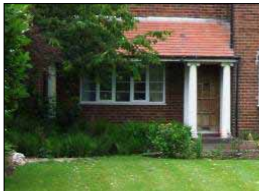
Photograph 11 (above): Example of columns
