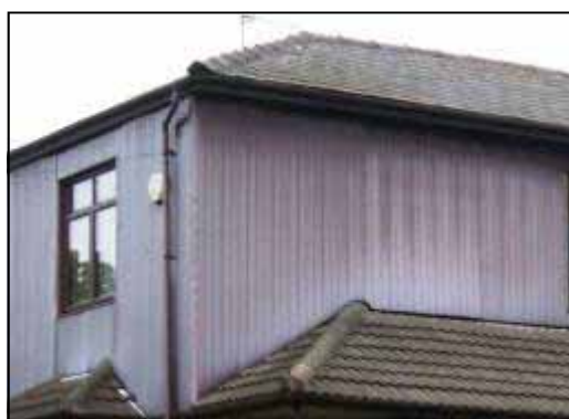
Photograph 12 (right): Timber upper floor.
