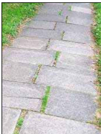
Photographs 20-1 (right): Examples of poor quality paving materials.
