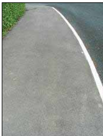
Photographs 22-3 (left): Examples of good paving surfaces.
