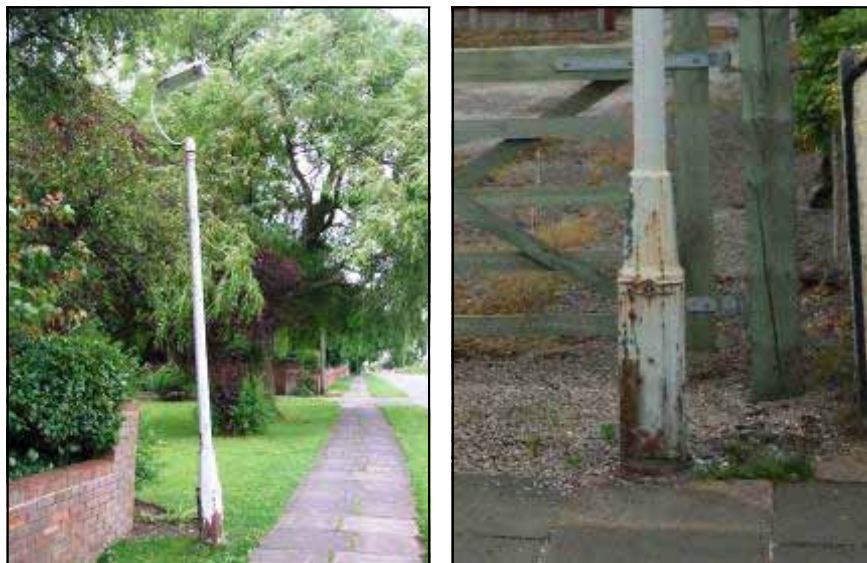
Photograph 24-5: Lamp posts found along Park Road. Interesting style but in need of maintenance.
