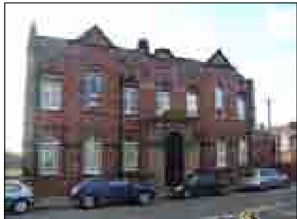
Photograph 17: front elevation of the Technical School building. Now converted into an adult education centre.
