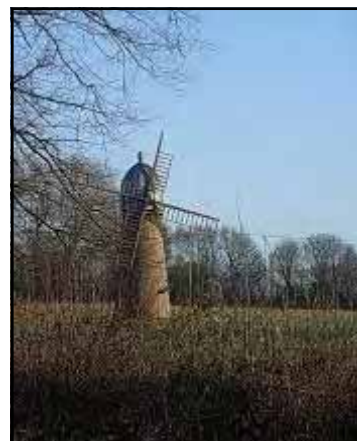
Photograph 45: Haigh Windmill as it stands today. In need of minor repairs.
