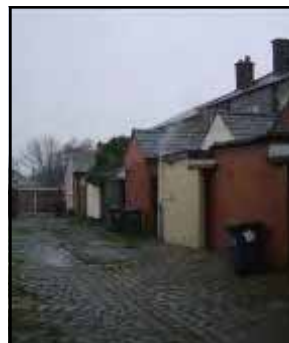
Photographs 37 & 38: Back lands of the two terraces found within the conservation area.
