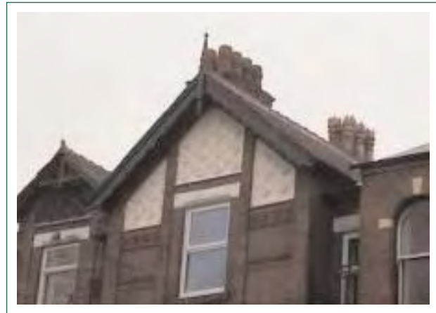
Detail of gable, No.16
