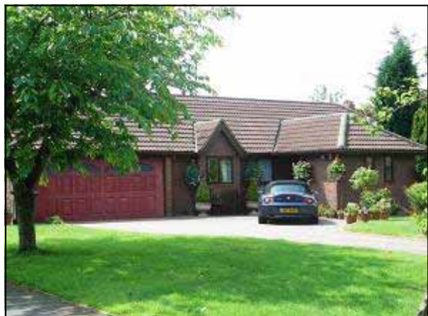
Photograph 25: Example of good quality infill development at Meadow Close
