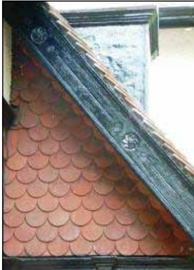
Photograph 26: Historic detailing on South Lodge, fish scale tiling and wooden barge board.
