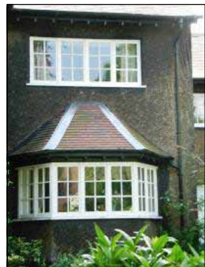
Photograph 12 (right): Example of bay window found in conservation area.
