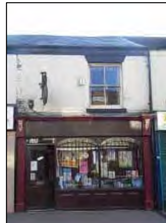
Photograph 20: Historic shop front at 14 Market Street
