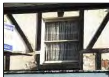
Photograph 40: Rotting wood
