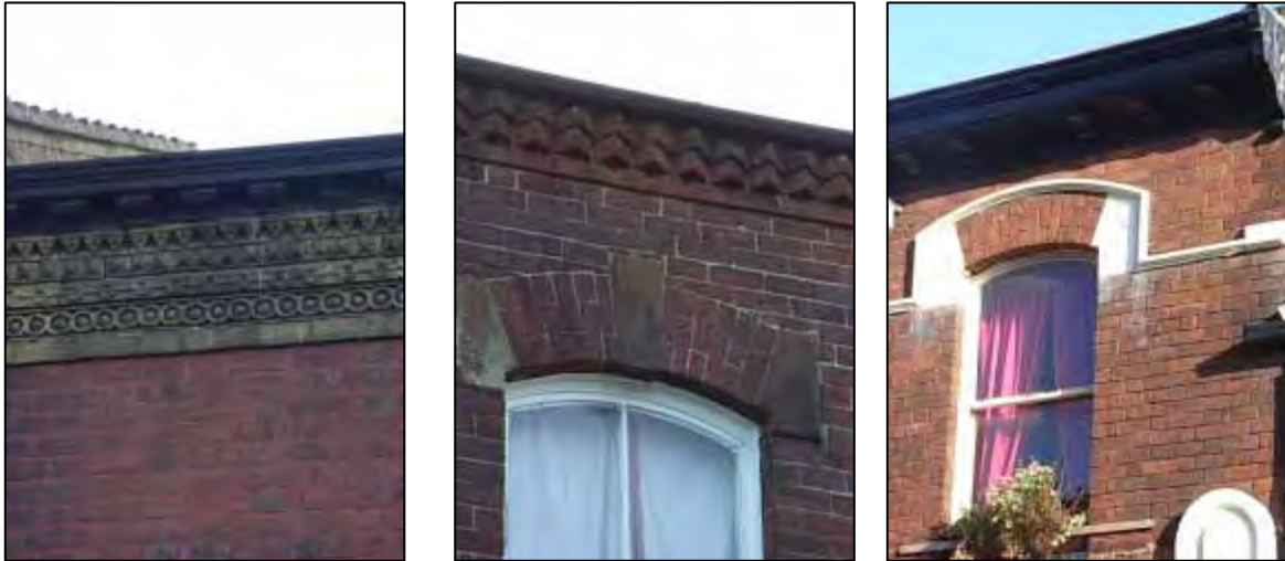
Photograph 8, 9 &10: Examples of Corbelling and window detailing
