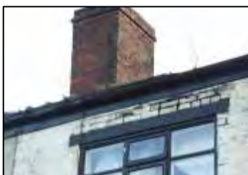
Photograph 38: Faulty guttering
