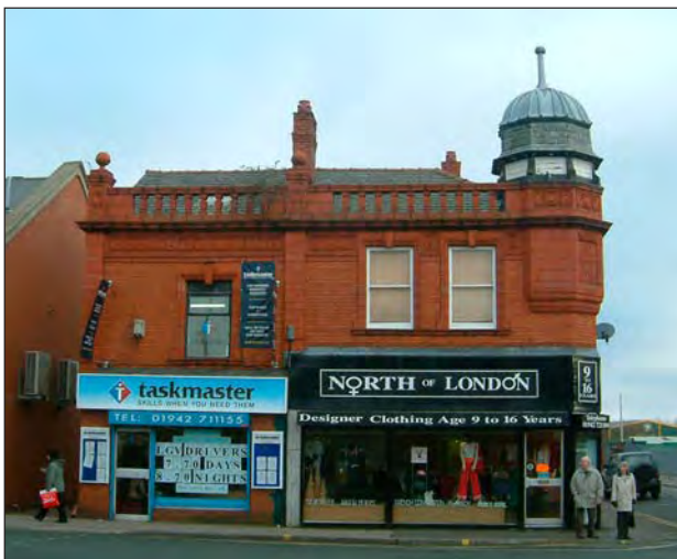
Bridge Foot House
