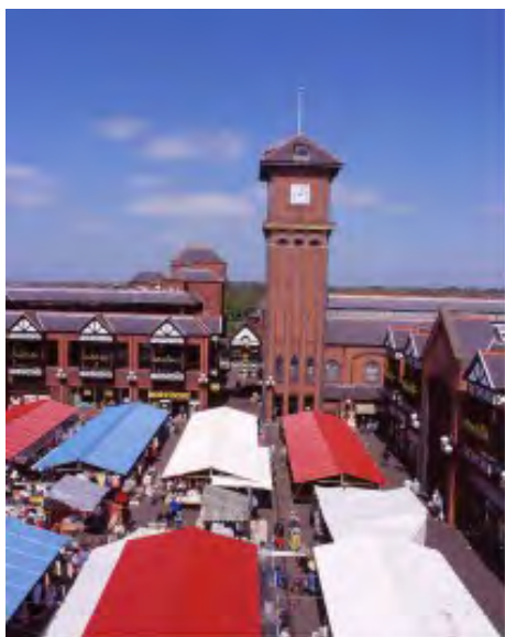
The Galleries Shopping Centre
