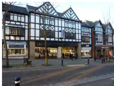
The Galleries Shopping Centre
