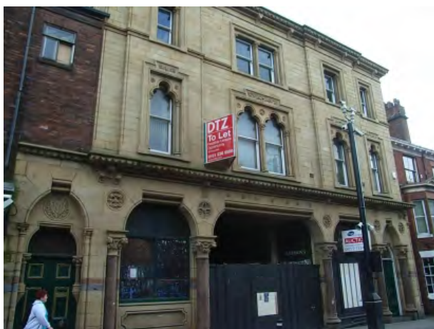
Grimes Arcade, King Street
