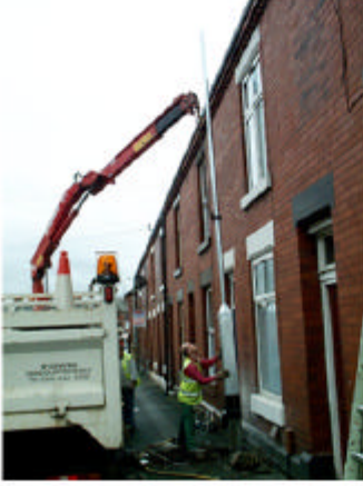
5. Slip new column over stump.
