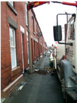
1. Support column & excavate base.
