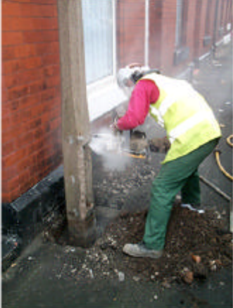
2. Cut column across top of door.
