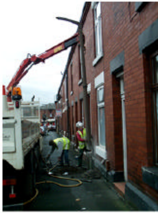
3. Remove top section of column.
