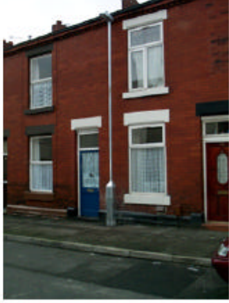
6. Connect up & reinstate to complete.
