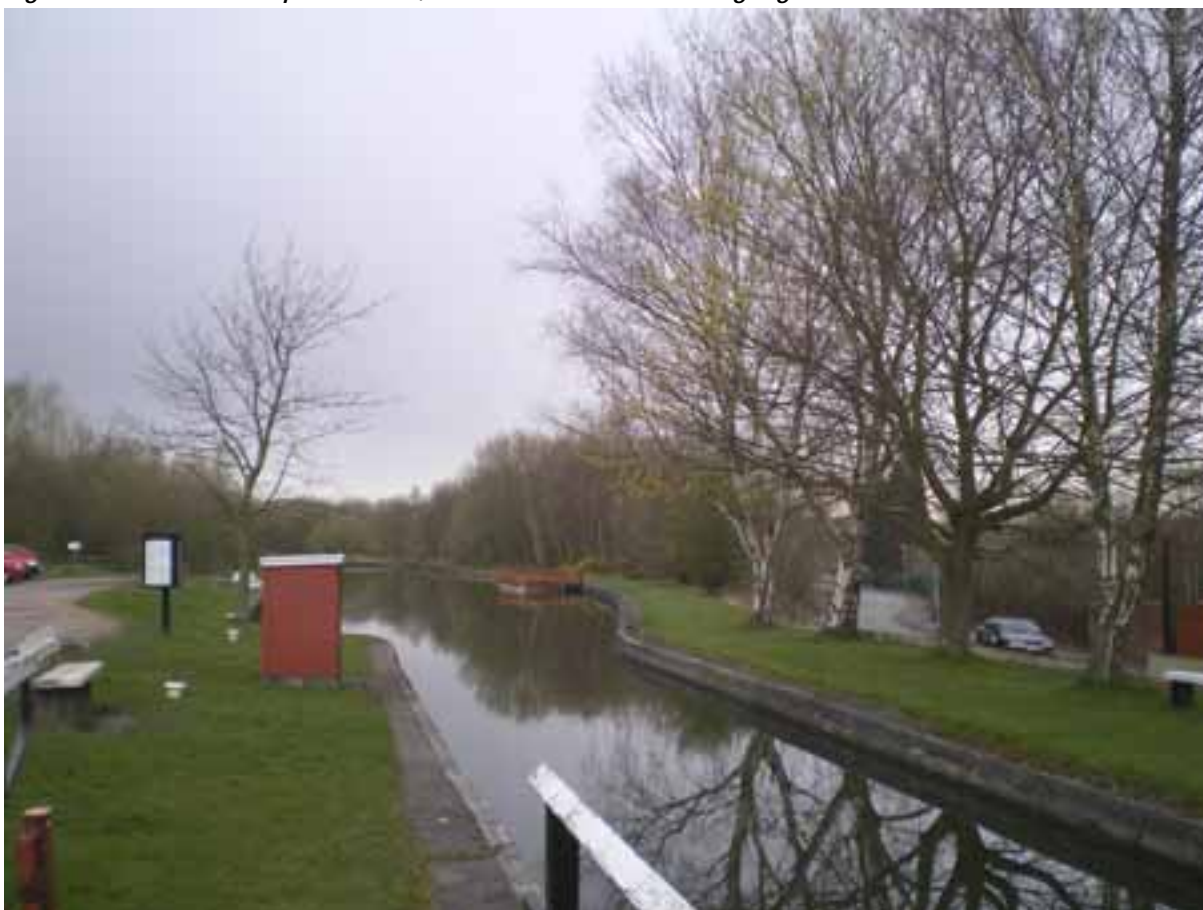
Figure 24: Leeds-Liverpool Canal, near Plank Lane showing significant modification
