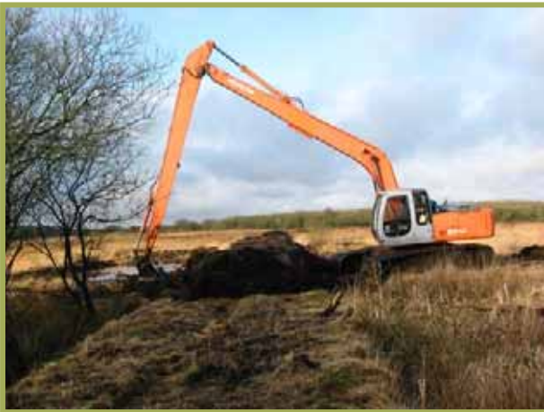
Bund heightening to isolate peat compartments
