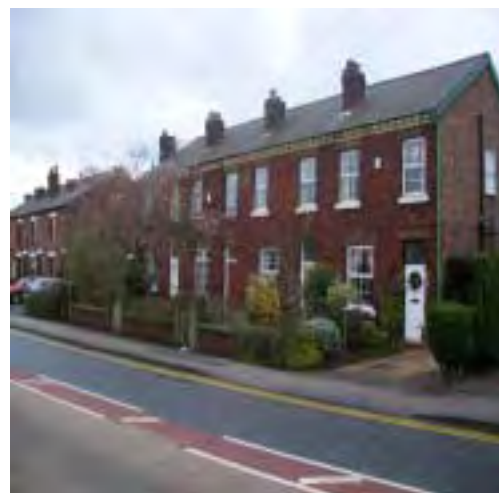
Later brick built terraces dating from late 19 th Century, (date stone in-situ)
