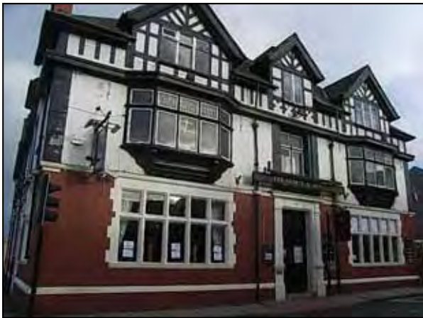
Photograph 16: front elevation of 185-7 Elliott Street, 'The George and Dragon' Public House
