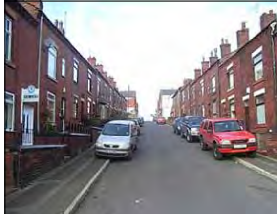
Photograph 44: View of terraced housing in proposed extension to the south-east of current boundary
