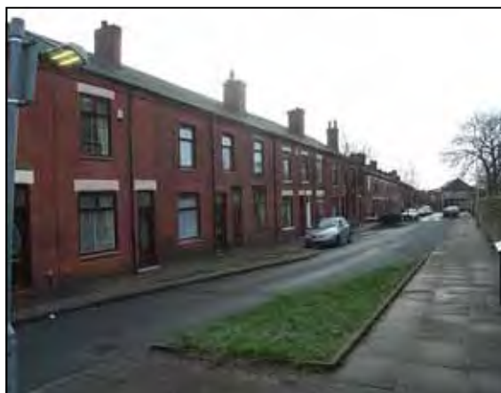
Photograph 39 (below): Row of Terraced housing along Saint George Street, in the proposed conservation area extension.
