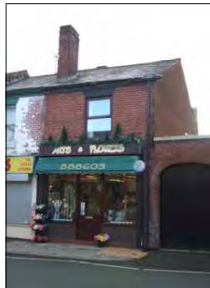
Photograph 21 (above): No 142 Elliott Street. An example of a high quality, sympathetic shop front within the conservation area.
