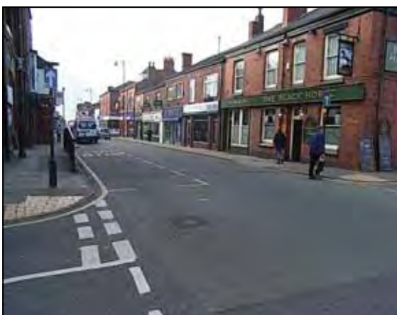
Photograph 43: View along Elliott Street showing some of the buildings in the proposed extension.
