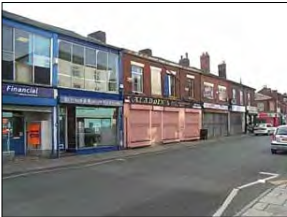
Photograph 22 (left): Metal Shuttering along section of Elliott Street.
