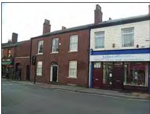
Photograph 12 (right): Front elevation of 138 Elliott Street
