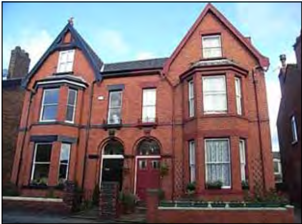
Photograph 14: Front elevation of 7-9 Upper George Street
