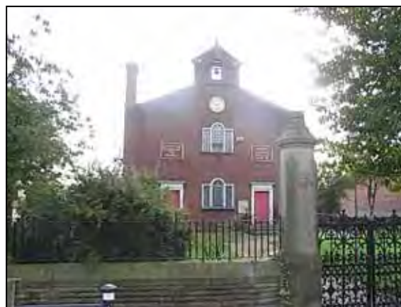
Photograph 10 (left): Side elevation of Top Chapel, showing current restoration works.
