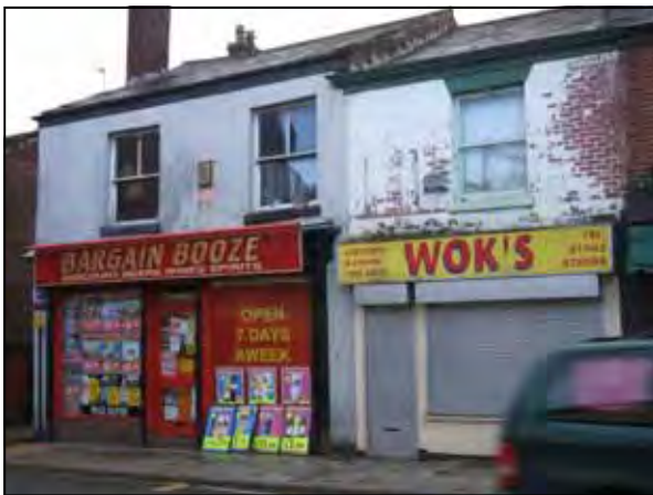
Photograph 20 (above): 144-146 Elliott Street. Examples of unsympathetic shop front design.
