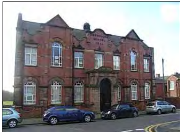
Photograph 17: front elevation of the Technical School building. Now converted into an adult education centre.
