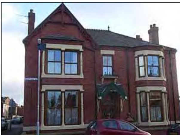
Photograph 15: Front elevation of No 13 Wareing Street, Tyldesley.
