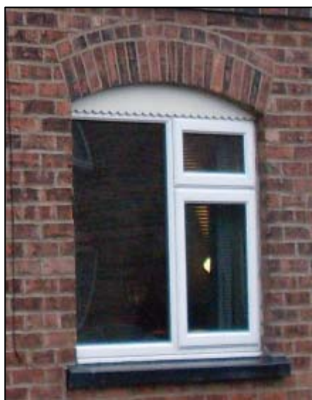
Photograph 13 (above): Example of an upgraded window frame
