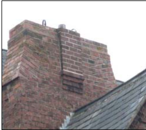
Photograph 10: Chimney detailing brickwork
