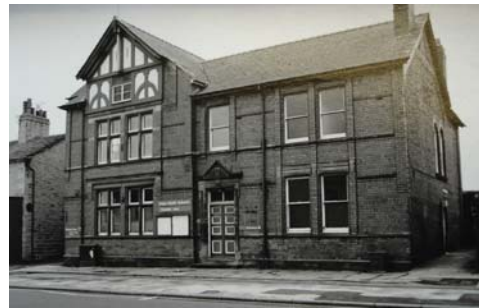
The Urban District Council Offices, High Street, demolished 1989, to be replaced by the Standish Clinic. Note the extended shopfront to Wellington Place, now a conservatory extension.
