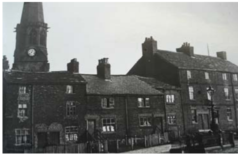
The cottages known as 'Spite Row', because local legend had it that they were built by Catholics to block the view of the Church.
