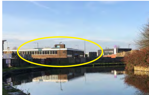
View of the ambulance station. The site is directly on the side of the canal and with being on a bend could have fabulous
