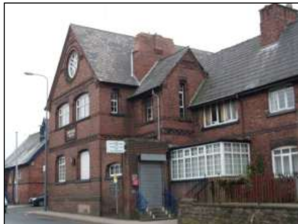
Photograph 9: Village Club, Leigh Road
