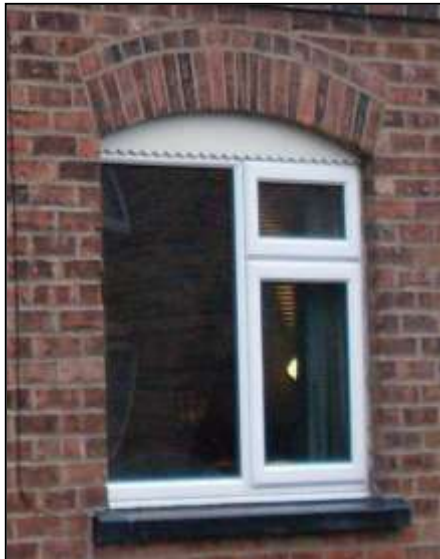
Photograph 13 (above): Example of an upgraded window frame
