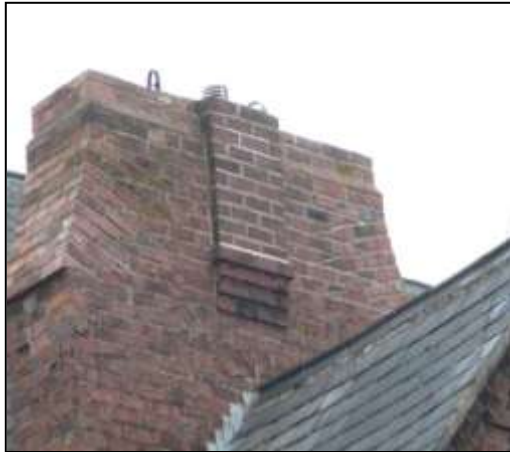
Photograph 10: Chimney detailing brickwork
