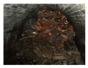
In urban areas consideration must be given to the need to provide alternative means to deal with flood water over and above that which can be accommodated by the culvert under design conditions. This will also provide contingency arrangements in the event of the culvert becoming blocked, and thereby minimising the risk of flooding to property.
