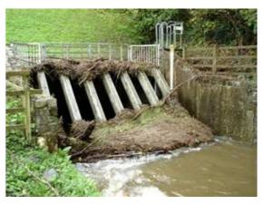
These screens themselves are often prone to blockage and require frequent clearance and robust emergency procedures in place to ensure that they do not in themselves cause, flooding.
