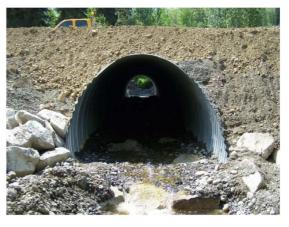
the lowered invert could be dressed with appropriately sized gravel. Actively introducing gravel will speed up the process of substrate replenishment, although velocities may need to be controlled to prevent washouts.
