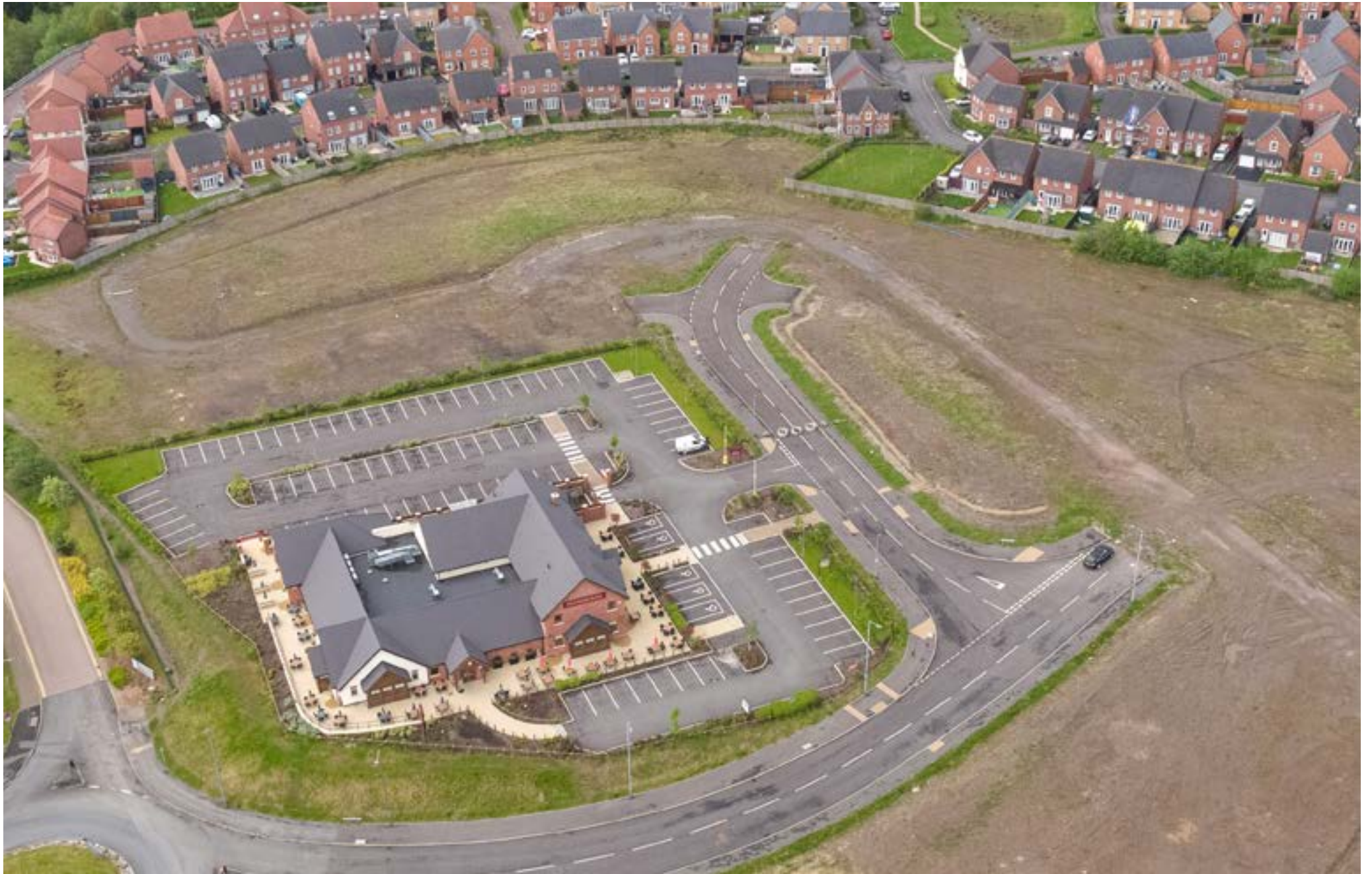
Smithy Brook Pemberton site - drone capture May 2021
