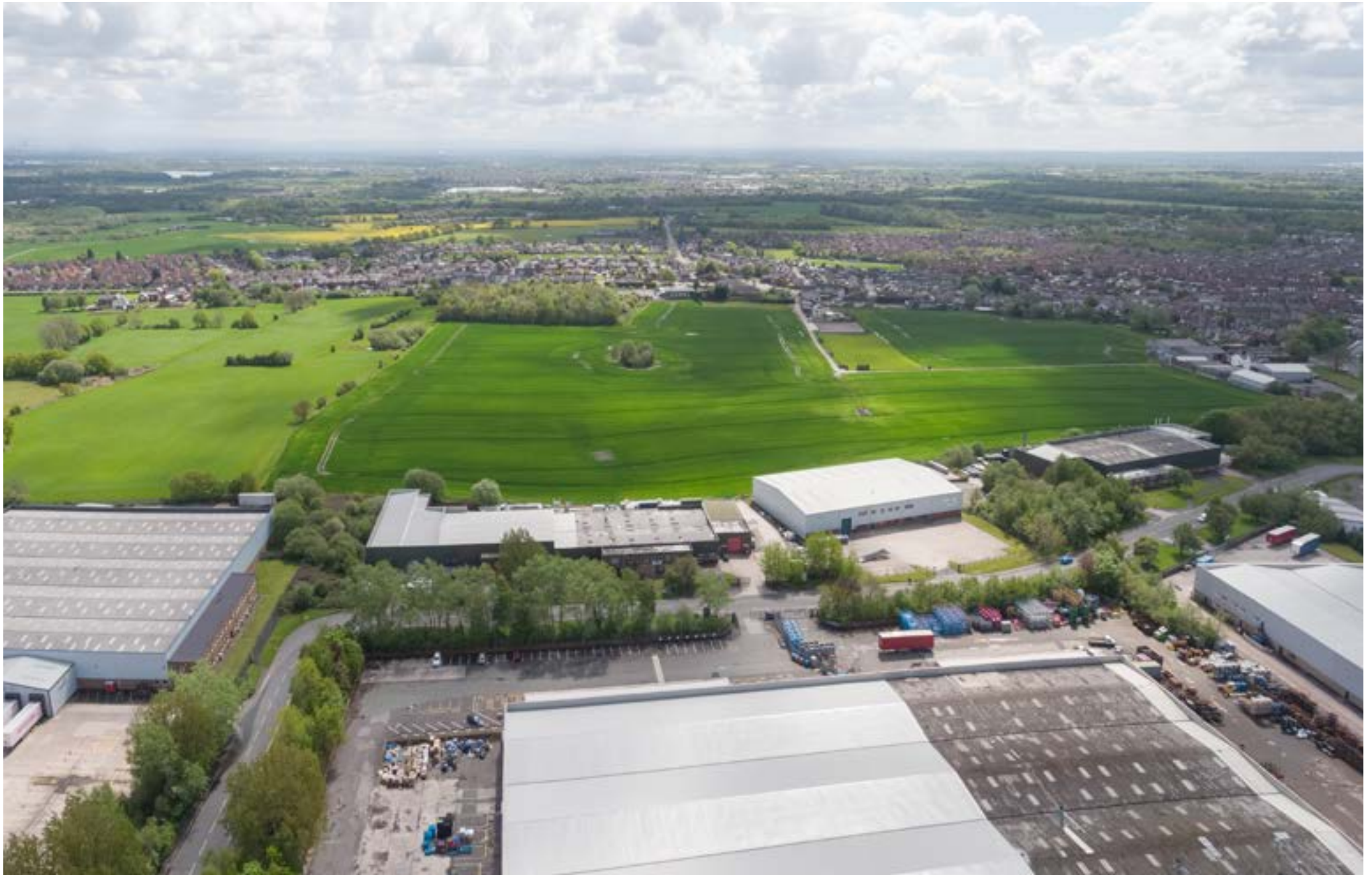
South Lancashire Industrial Estate Extension - drone capture May 2021
