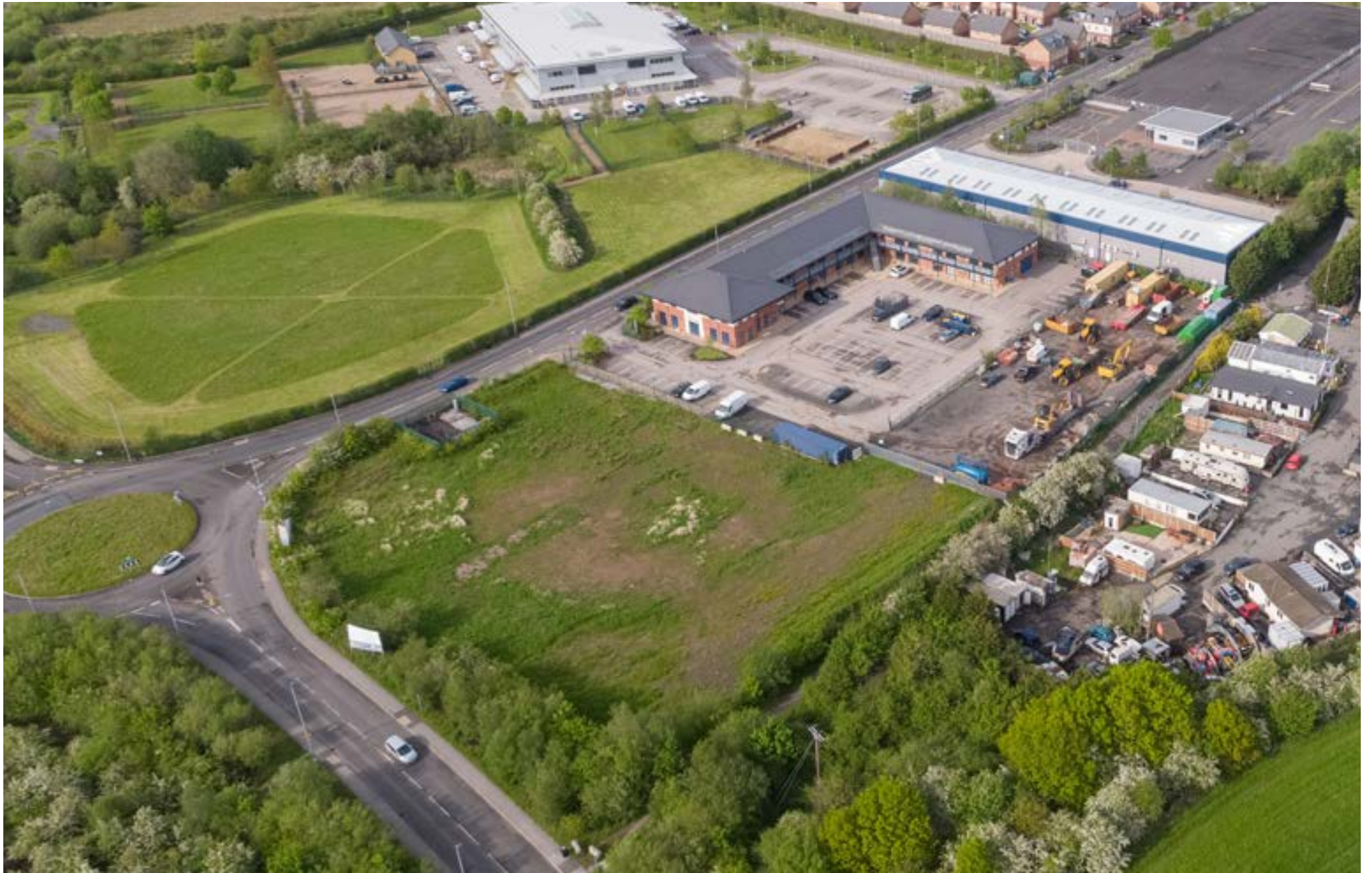
Gibfield Park (Plot 2) - drone capture May 2021
