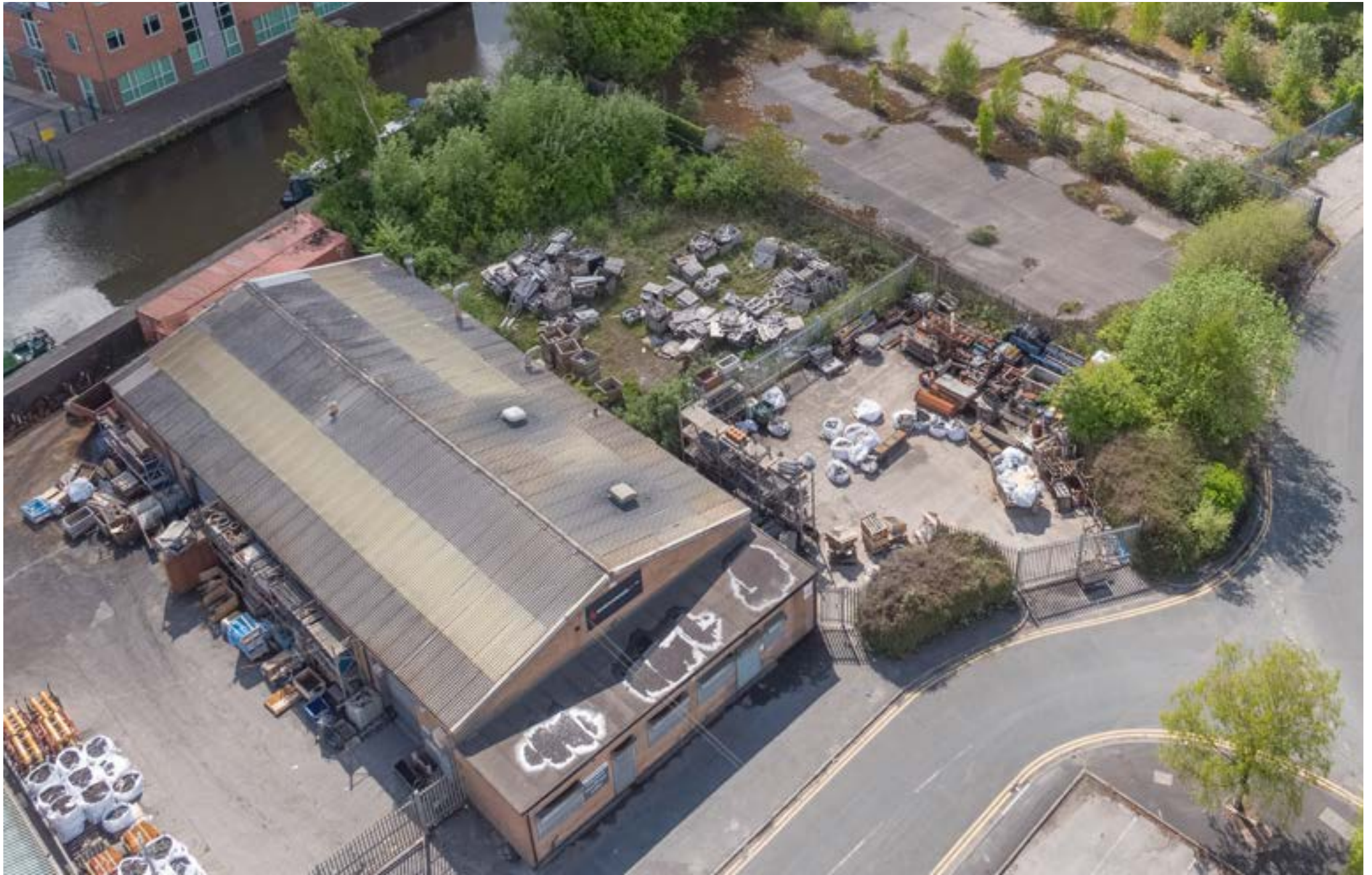
Wigan Pier Quarter, Plot 2 - drone capture May 2021
