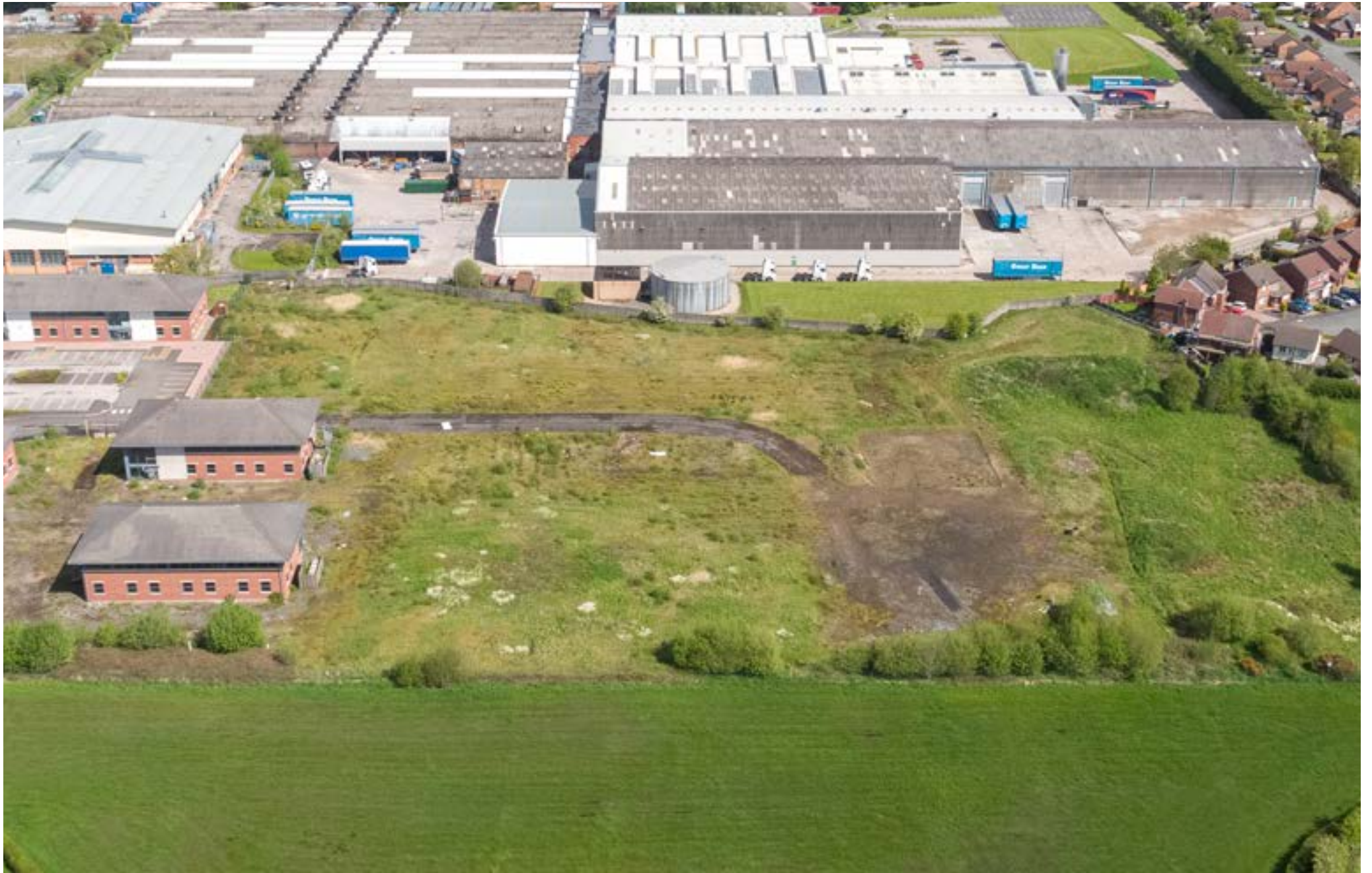
Warrington Road (Plot 3) - drone capture May 2021
