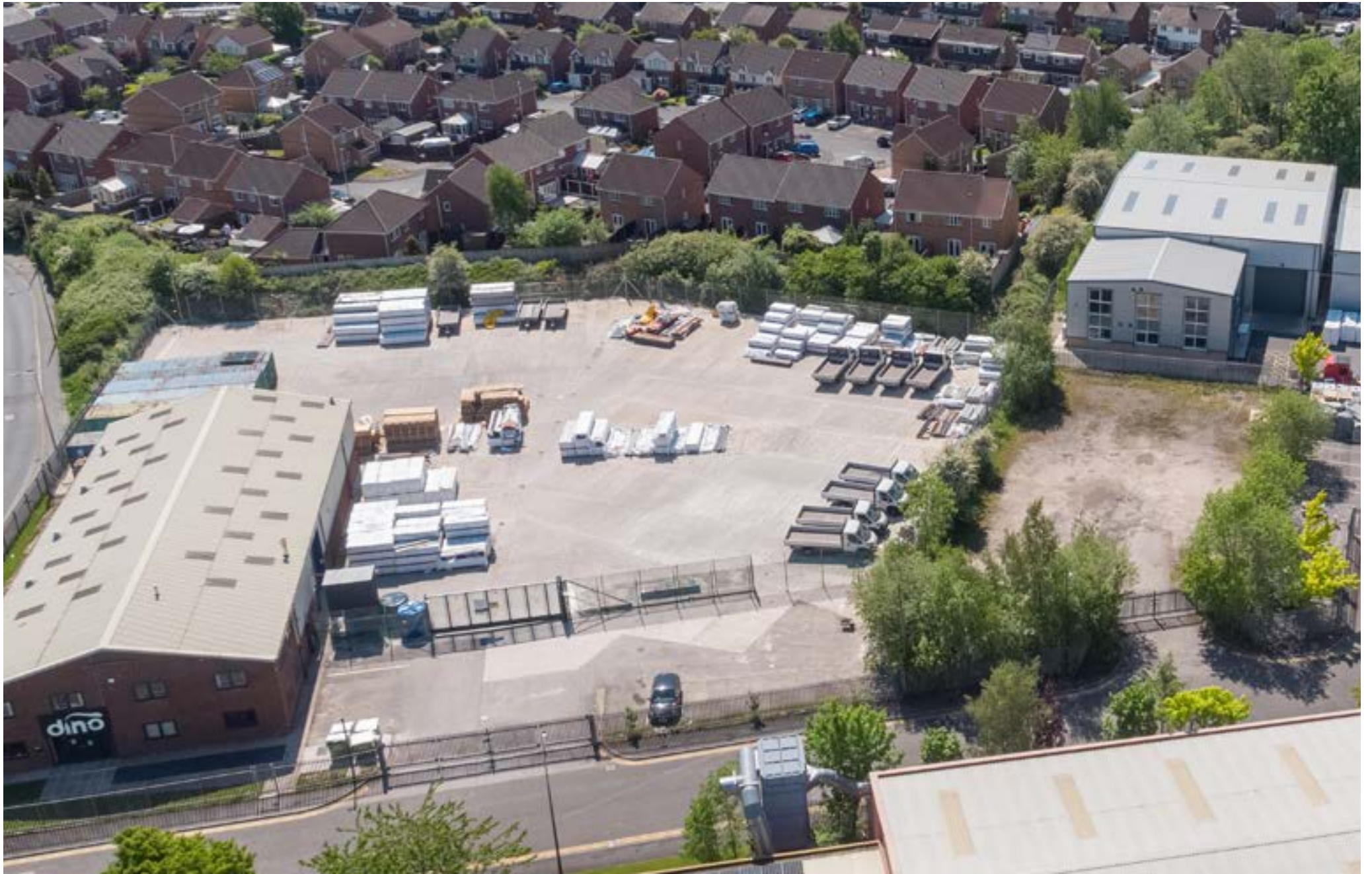
Swan Lane (Plot 2) Hindley Green - drone capture May 2021
