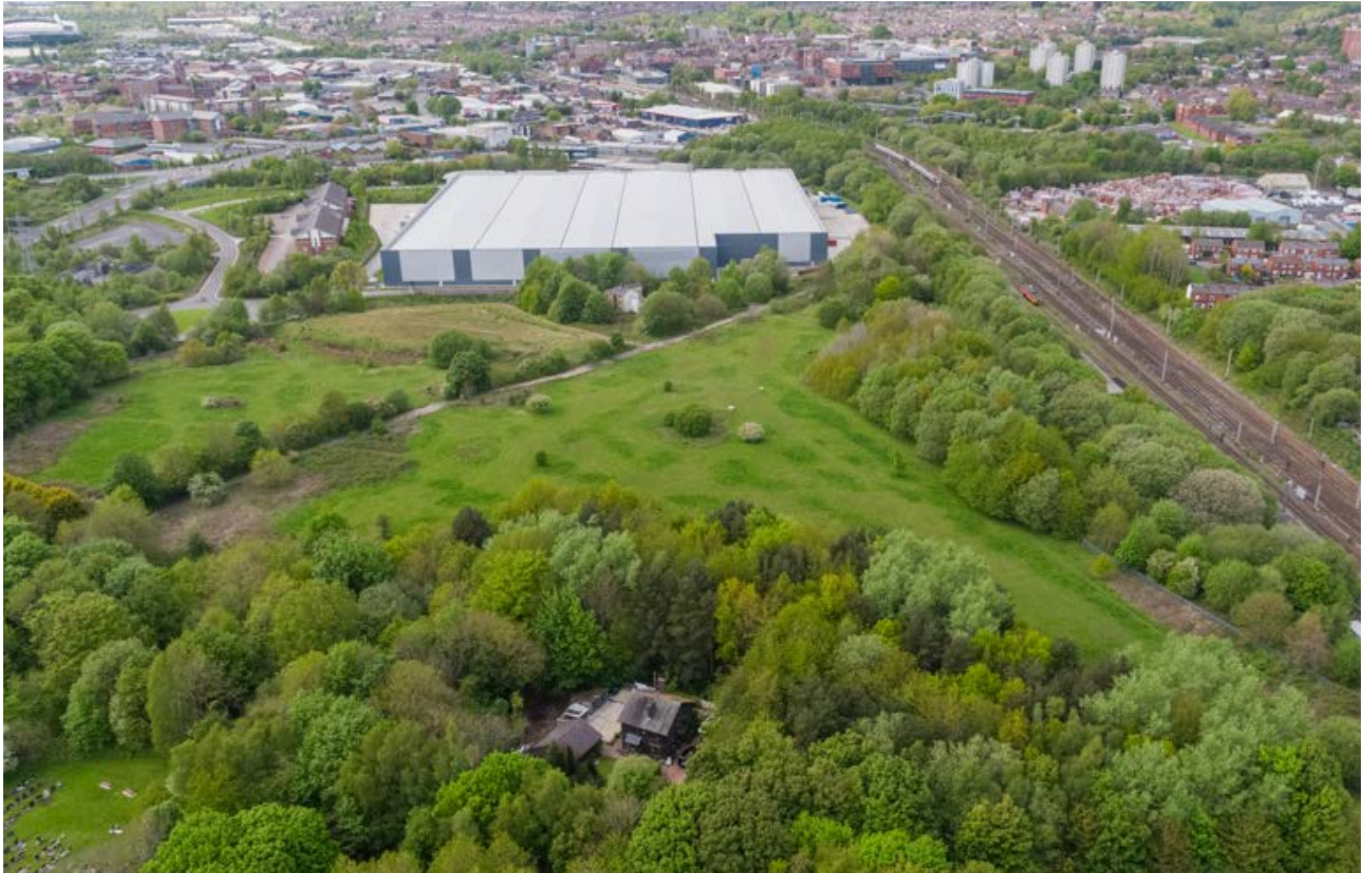
Westwood Park site - drone capture May 2021
