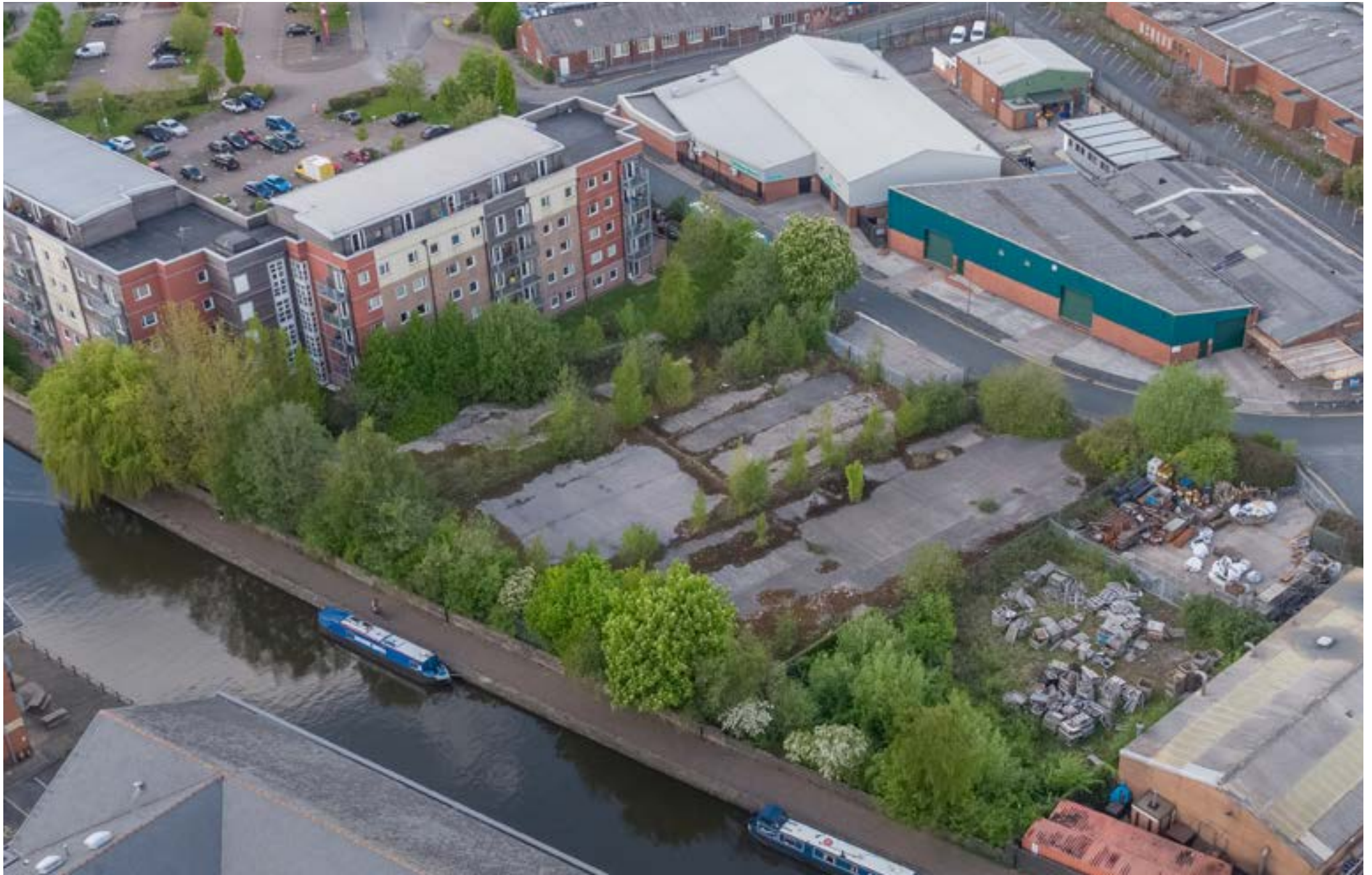
Wigan Pier Quarter Plot 1 - drone capture May 2021
