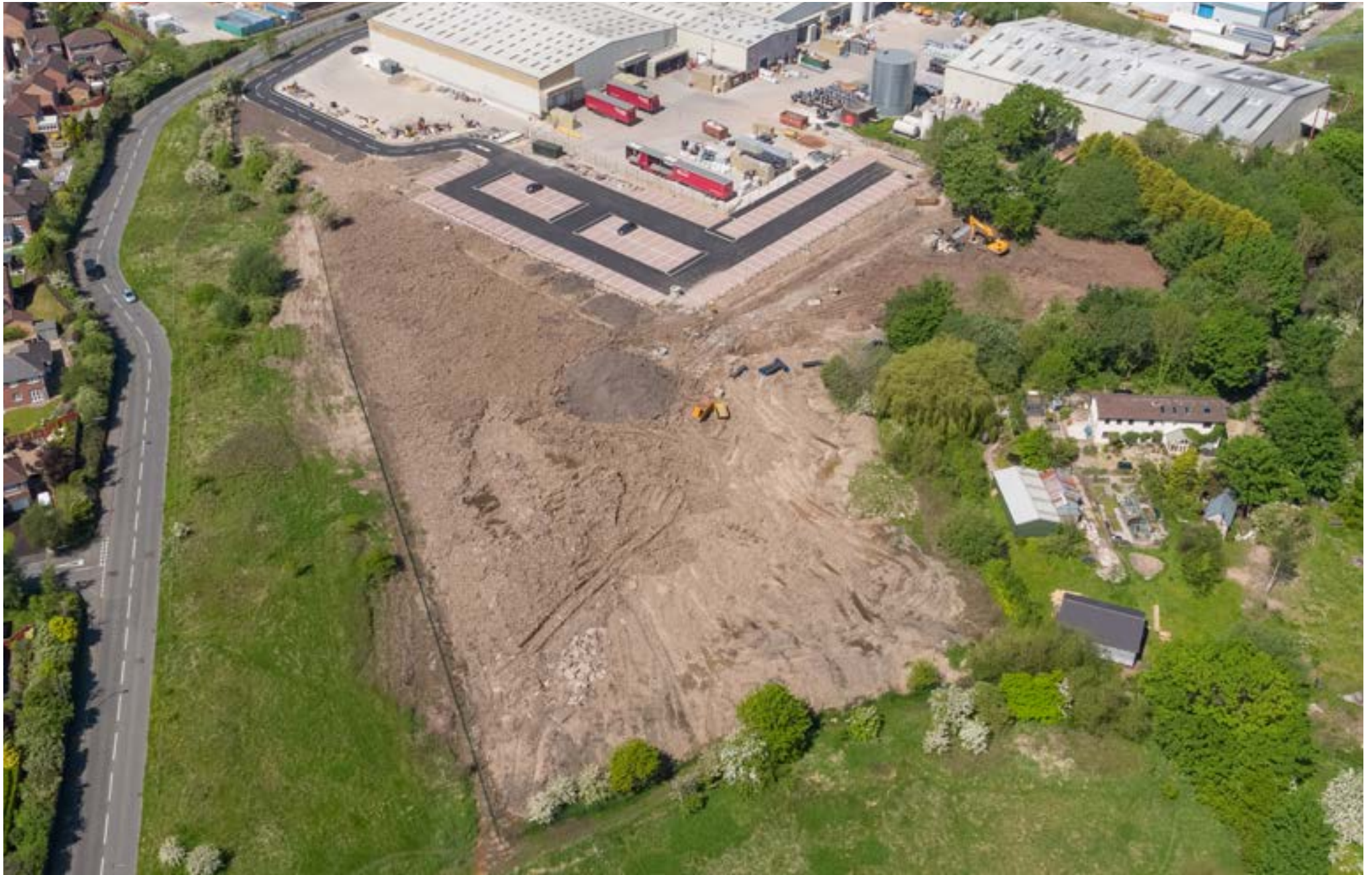
Swan Lane (Plot 3) Hindley Green - drone capture May 2021
